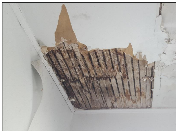
Photo 1: The moldy boards inside Arika's ceiling
