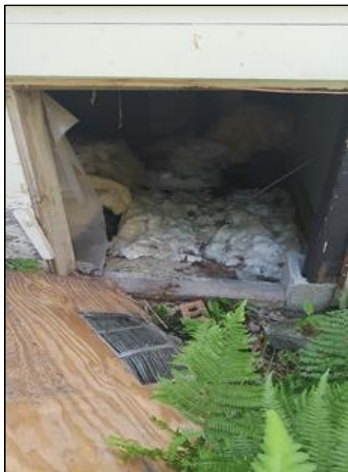
Photo 2: Behind the loose panel under Dawn's building
